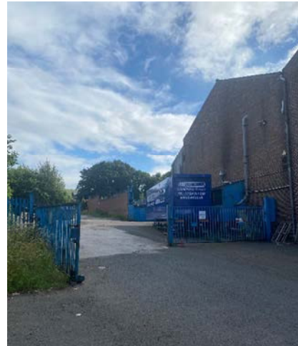
Side view of Engenda Manufacturing Plastics Unit with access and hard standing
