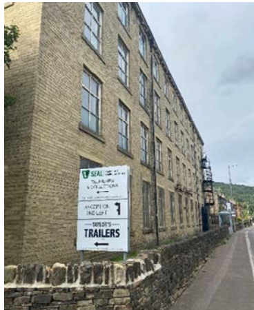
Mill building fronting Park Road
