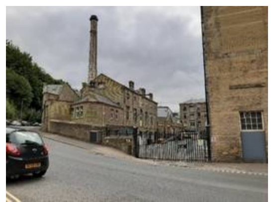
Mechanics Workshop buildings
