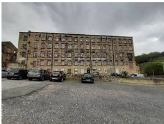
Across site to Stone Dam Mills
