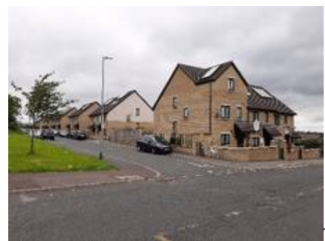
Residential development Vickerman Street
