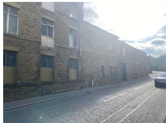
View of vacant buildings on site (Dewsbury Road) which will be demolished for redeveloped to residential
