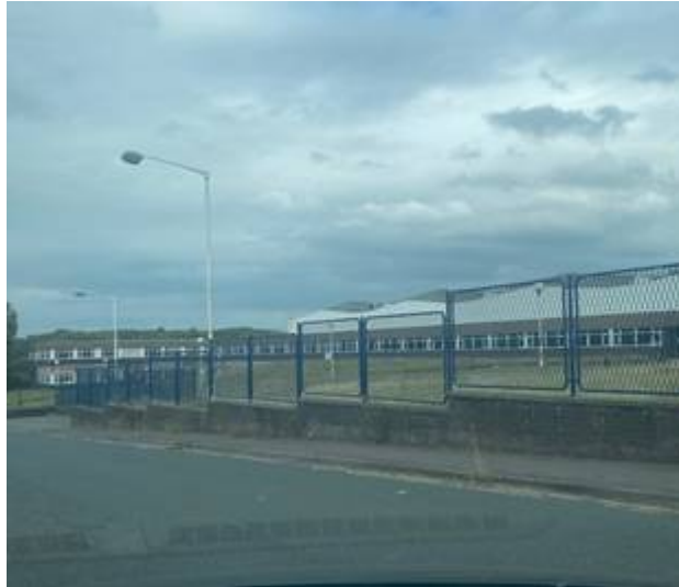
View of the site from entrance off Brighouse Road
