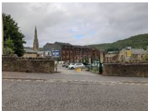
Across New Road towards Deal Street
