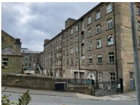
Mill buildings rear elevation
