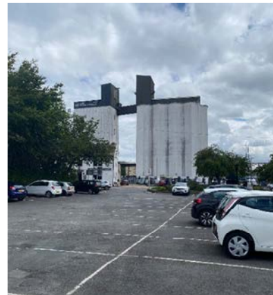
Daisy Street Car Park with ROKTFACE climbing wall in the distance
