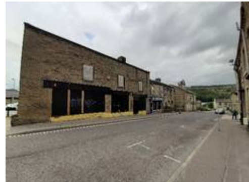
Empty units New Road
