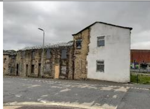
Dilapidated buildings Hopwood Lane
