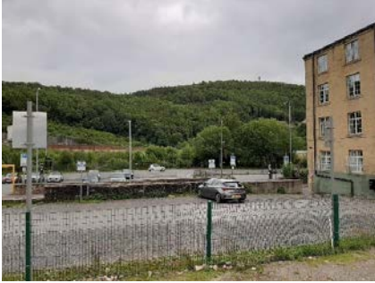
Looking east across the site
