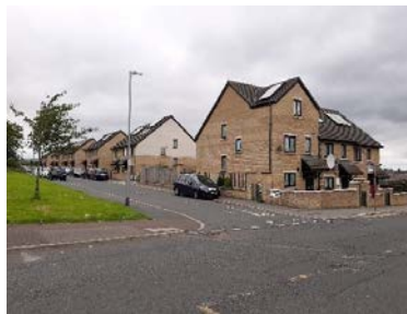
Residential development Vickerman Street
