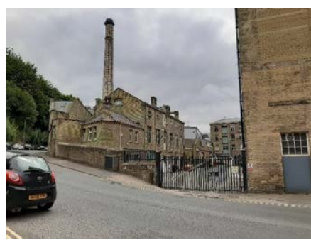
Mechanics Workshop buildings
