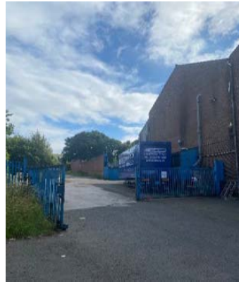
Side view of Engenda Manufacturing Plastics Unit with access and hard standing
