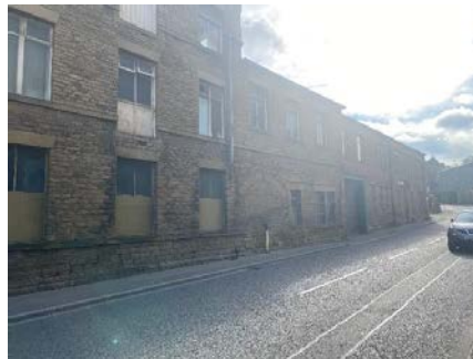
View of vacant buildings on site (Dewsbury Road) which will be demolished for redeveloped to residential
