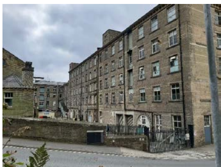
Mill buildings rear elevation
