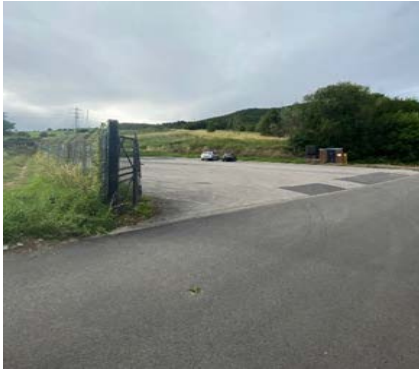
Car parking and hard standing at rear of the site
