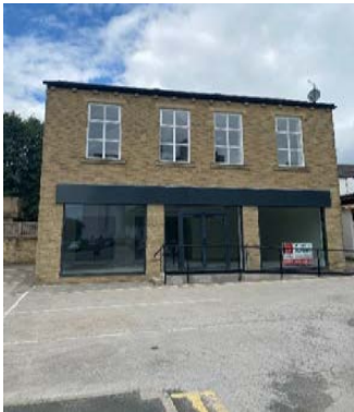
View of 1,567 sqft newly refurbished retail unit in Daisy Street Car Park available at £15.95 psf (£25,000 per annum)
