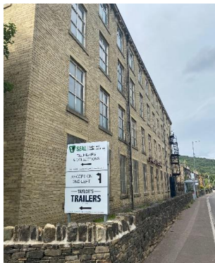
Mill building fronting Park Road
