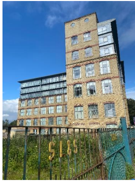
Mill building converted to residential adjacent to the site off Dewsbury Road
