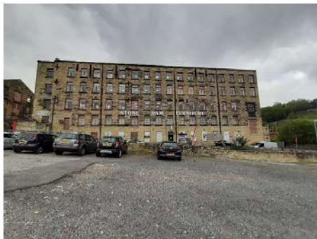
Across site to Stone Dam Mills
