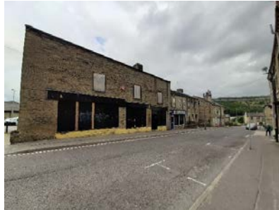
Empty units New Road
