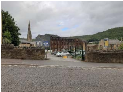
Across New Road towards Deal Street
